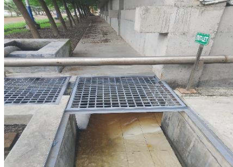
Sampling point surrounding environment 06/10/2024
