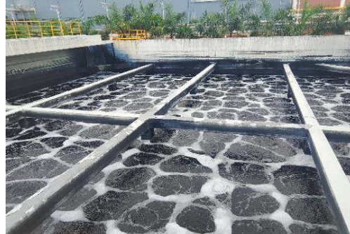
Sampling point surrounding environment 06/10/2024
